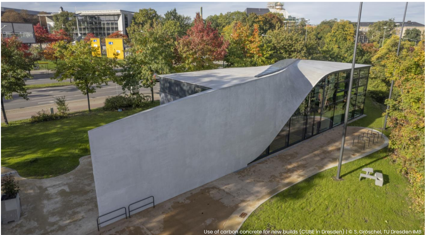
Use of carbon concrete for new builds (CUBE in Dresden) | © S. Gröschel, TU Dresden IMB
